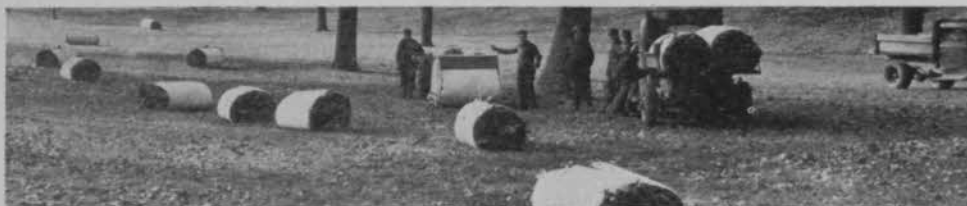
1947 Field demonstration of the 45" Parker Fairway Sweeper shows bales of leaves which have been swept up by one-man operation at the rate of 500 bushels per hour. The sweeper collects the leaves in bales holding approximately 25 bushels which are easily transferred by truck to compost pile or disposal area.
