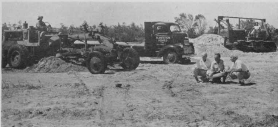
Chauncey R. Clark (center) and Stewart E. Clark (R) who head up Plantation Homes, Inc., listen as Robt. F. "Red" Lawrence points to outline of fairway under construction on new golf course. Latest earth-moving machinery shown in the background will help make it possible to complete construction in record time.
