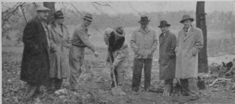
Glen Head CC pres., Jay Gilman, breaks ground for $100,000 addition to clubhouse. L to R: Robert Grieve, Peter Reiss, Charles K. Howard, Jay Gilman, Irving Spanier, Dr. Michael Berliner, Fred Grieve.
