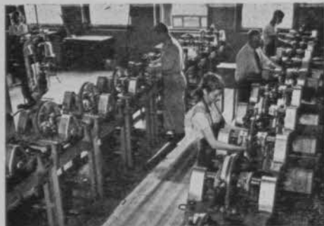
Semi-automatic golf ball winding machines electrically controlled stop at pre-determined size thus speeding up production. The machines stop automatically in the event the rubber winding thread should snap.
