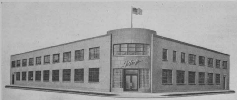
Golcraft's new and modern plant is at 1700 West Hubbard St., conveniently located near downtown Chicago.
