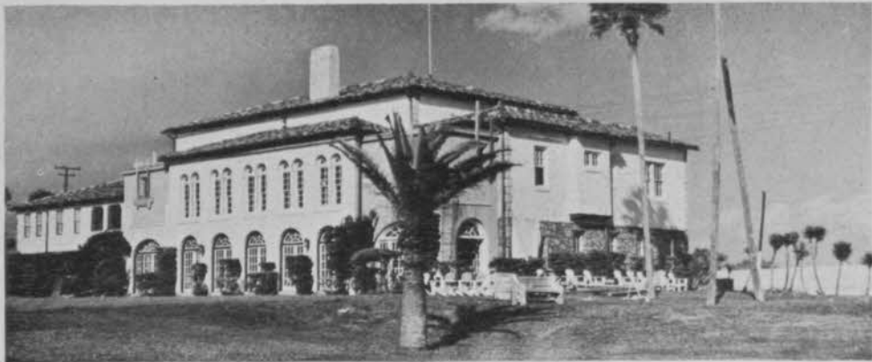
Seabreeze clubhouse renovated inside and out for reopening after wartime shutdown.
