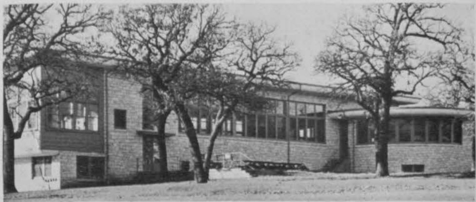
The recently completed $85,000 NTSC recreation building and clubhouse extends a welcome to golfers and party groups. Golf shop and lockers are on the basement floor. Solarium is at the left, the main room is for recreation and the rounded section houses the snack bar.
