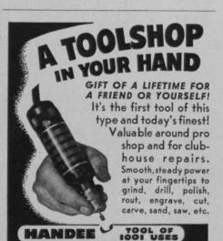
The efficient Handee works on metal, alloy, plastic, wood, horn, bone, glass, etc. 25,000 r.p.m. AC or DC. Easy to handle. Weighs only 12 ozs. GET THE HANDEE KIT. A handsome, all-steel case with Handee Tool and a complete assortment of 40 accessories. Complete, \$27.50. Handee only, with 7 accessories, \$20.50. Get it at stores everywhere. If they can't supply you we'll send it postpaid. Satisfaction Guaranteed! Free — New 52-page Manual.
