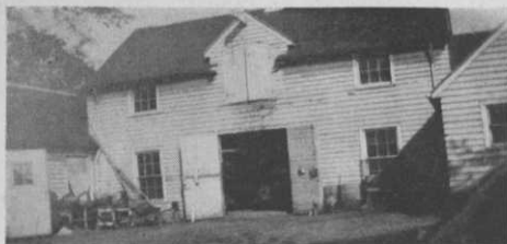
Yard front of Oakwood equipment building.
