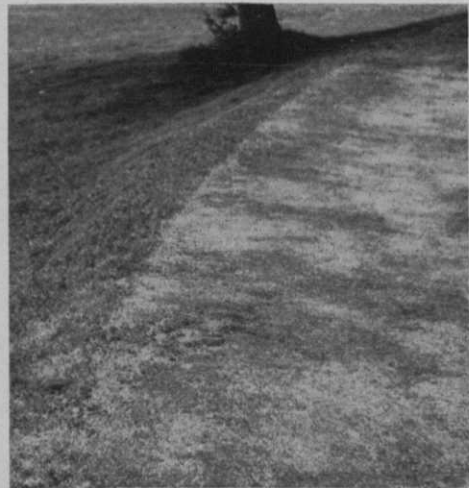
Abrupt banking around edges of green sheds water and dries the soil in the green
