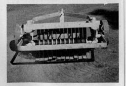
Illustration shows cultivating position. Weights on tray over axle regulate depth of cut. Circular knives made of fine knife steel. A real machine.
