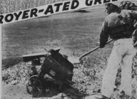
A Royer Model "K" turns out 3 to 6 cu. yds. of compost per hr. for Sugar Creek Golf Club, Ohio.
