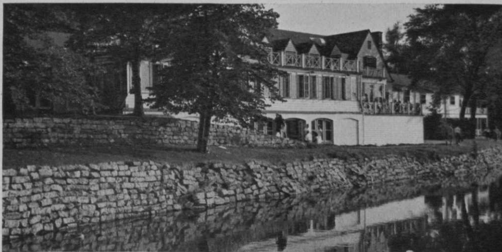
"Before" view of Tam O'Shanter clubhouse shows conservative English Tudor style architecture which prevailed before building was redesigned.
