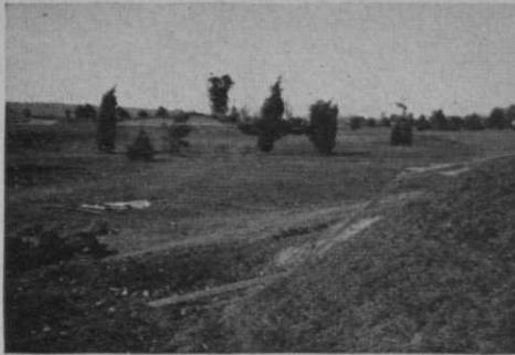
Fig. 3—Note how gauge shows bed-knife lines of gang mowers, in determining how bank should be regraded.
