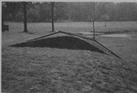
Fig. 1—Original grading at top. Note how regrading gauge shows where gang-mower cut would be. The stick extending from center section is folding rule opened to 5 ft. to show center section length.
