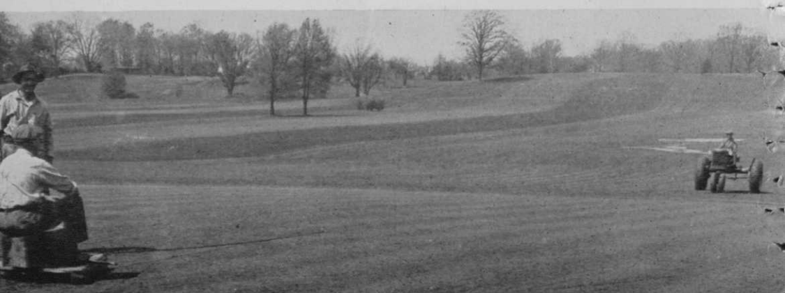
Fig. IA.—A tractor, moving backwards draws and helps to guide the turf cutter across the green.
