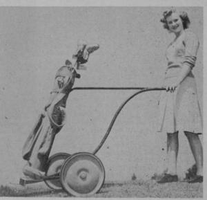
KANGAROO KADDY FEATURES: double-ball-bearing wheels, wide-spread for balance on hillsides. Lightweight, fingertip balance. Built of chrome molybdenum steel tubing, electrically welded. 12-inch wheels. Wide rubber tires will not cut greens.
