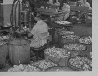
factory, a special reclaiming process goes to work to recover the usable rubber. The illustration shows a workman removing covers after the old balls have been sorted into types. To make sure that the remade balls measure up to the high standards set, a compression machine checks hardness before they are shipped.
