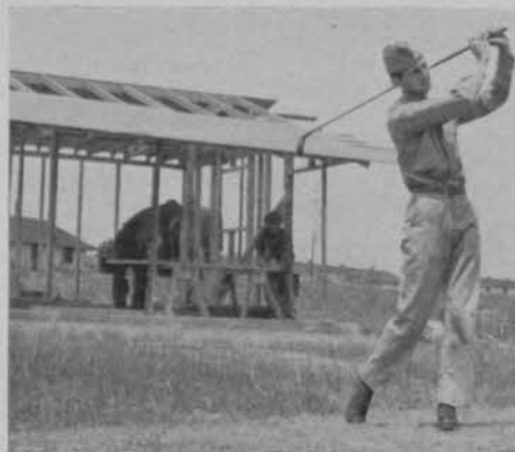
Pvt. Fred Johnson, formerly at Philadelphia Cricket Club, on the golf practice range at Camp Croft. In the background is the range golf shop being built by soldier-carpenters.
