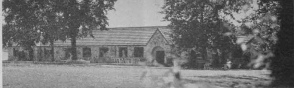
Front view of Walnut Grove's attractive clubhouse, which overlooks the first tee and eighteenth green. Additions were made to the structure in 1936, '38, '40 and '42.
