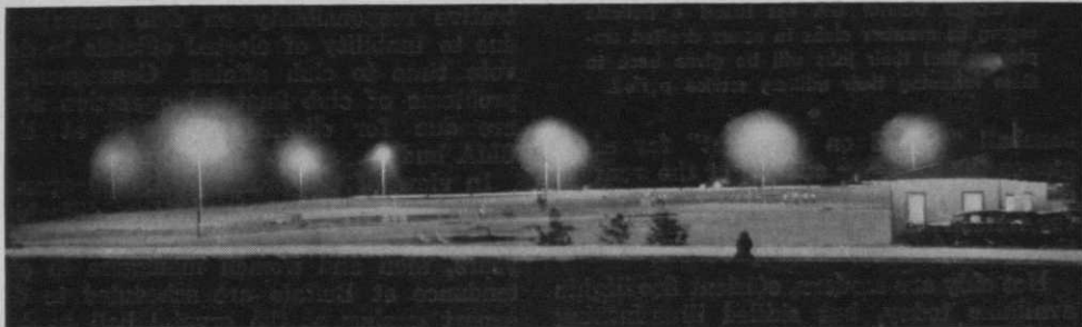
Business boomed at this 14-acre pitch and putt golf practice course when 33 1,500-watt floodlights were installed.
