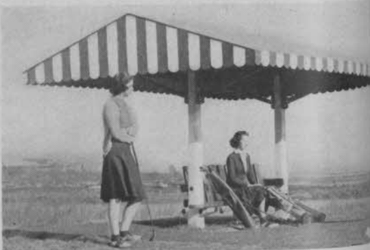
Both seat and roof of shelters in use on course at the U. S. Navy Yard, Charleston, S. C., are supported on a pair of reinforced posts. The roof is of wood, painted to simulate a canvas awning.
