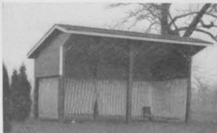
Shown above is the new practice driving shed constructed this year at the Whitmarsh Valley CC in the Philadelphia District. The cost of the shed was around $300, according to Pro Morrie Talman. Morrie is now able to give lessons at any time, rain or shine, and can also provide an added bit of privacy for students taking lessons from him. The practice shed has been 'well worth the cost,' Morrie says.
