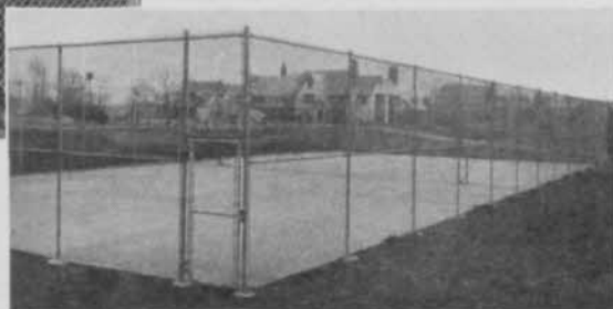
Another view of chain link fence, used to enclose tennis courts on private club grounds. Note the metal posts set at 10-foot intervals in bell-shaped concrete footings.
