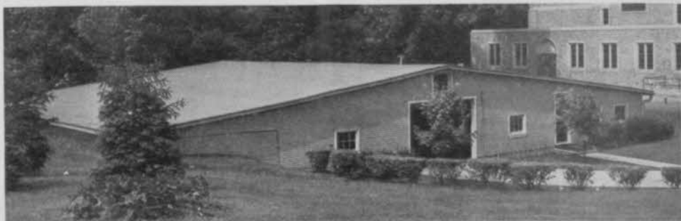
How is this for an equipment and tool barn? Originally an old shed, Notre Dame spent $3,000 to modernize it for maximum greenkeeping efficiency.
