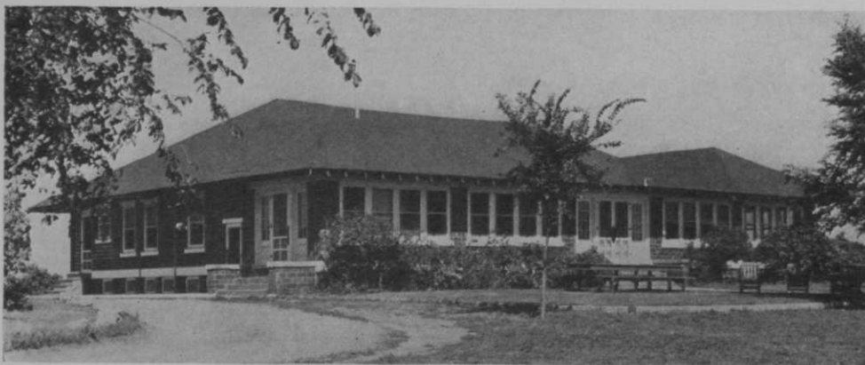
A new heating plant installed this spring will now enable Spencer CC's members to make use of their compact, newly remodeled clubhouse the year-round.
