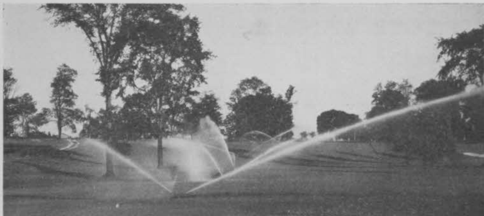
A fairway watering system is not for every-day use; rather, it serves as insurance against baked turf during protracted dry spells.
