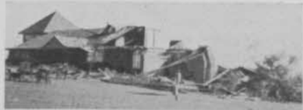
At Leicester, Mass., the hurricane demolished half the clubhouse.
