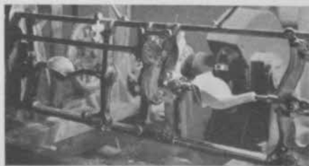
The blocks are then "roughed out" by this lathe, which automatically follows a master pattern.
