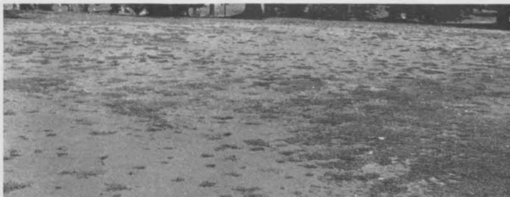
Remains of what once was a fine putting surface. Damage occurred under climatic conditions not found in Northern summer resort areas.
