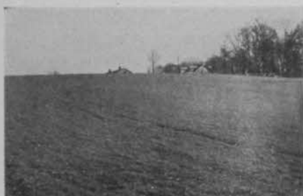
Amount of clearing needed is suggested by these before-and-after 7th fairway photos.
