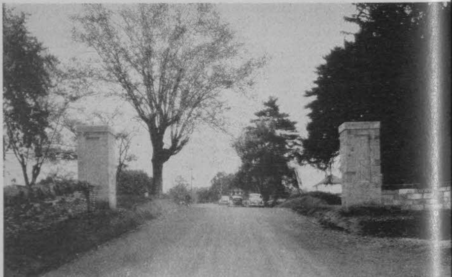
Since Bedford is the "Stone City," the attractive entrance pillars to Otis Park are appropriate of native limestone.
