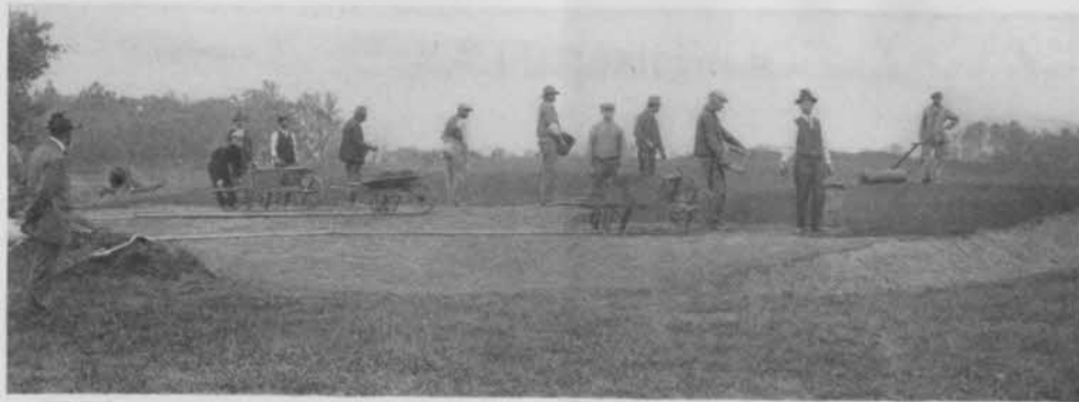
Dr. Harban (extreme left) watches workmen applying creeping bent stolons to a putting green of a private course—the ninth at Columbia CC, Washington, D. C., 1919.
