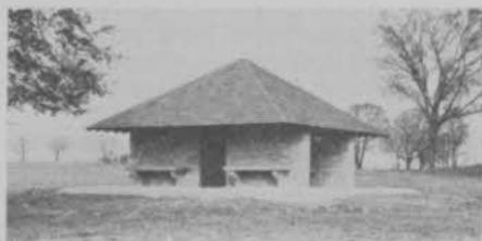
One of several shelter houses built for convenience of O.S.U. golfers.
