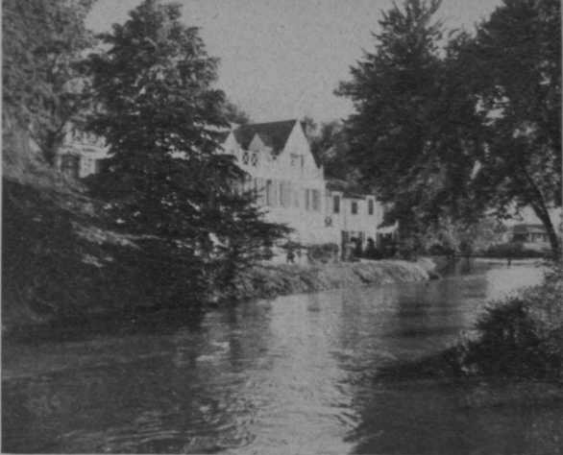
When fire destroyed the clubhouse of Tam O'Shanter CC (Chicago district) last fall, the club promptly laid plans for a replacing building. Here you see it as recently completed; its interesting site is along the upper reach of the Chicago river.
