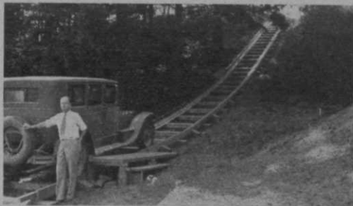
This motorless, cable-drawn auto lifts golfers to the next tee 70 feet above. Length of slope, 215 feet.
