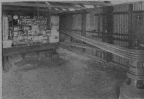
Here a deep well pump has been powered with the Diesel engine for economy.
