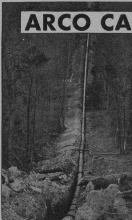
(Above) Note the adaptability of the flexible coupled line to the contour of the ground.
