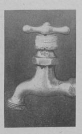
closing of the valve is of course commonly done, but that is the way a good many handles and holding screws become lost and misplaced when badly needed later on. The photo shows a simple way to block a tap open, proof against everything but maliciousness.
