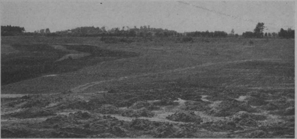
Topsoil on No. 9 green at Portland (Me.) municipal course before spreading. No. 1 fairway at left being disced
