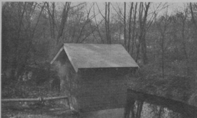
This pumphouse, on the banks of Kyte Creek, cost only $250 to build.
