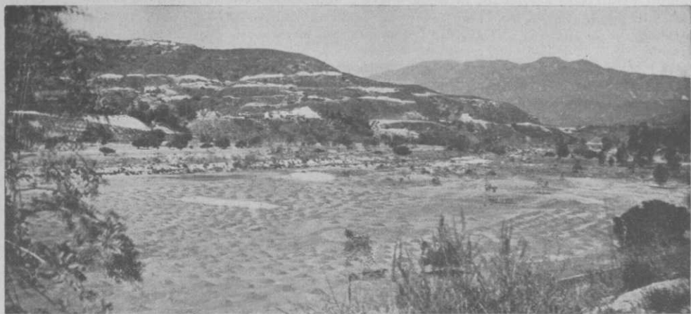
A new 9-hole golf course is being built in this old river bed at Pasadena. The piles are topsoil to cover the sandy bottom
