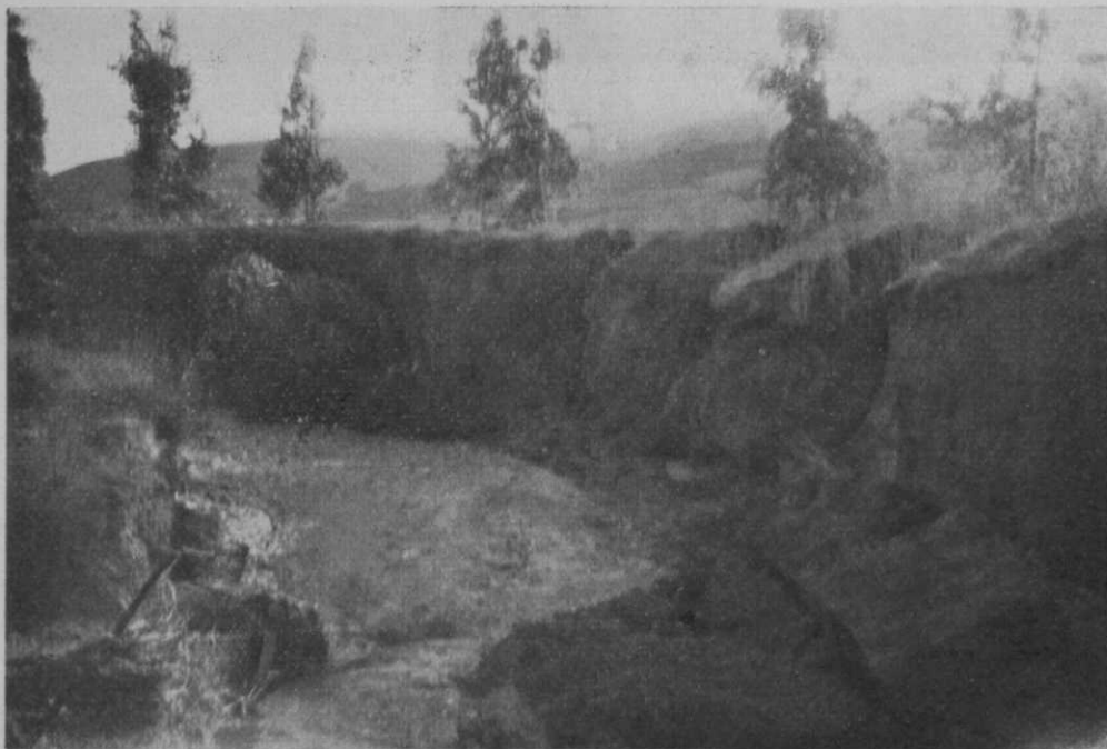
How storm waters destroy in California. Newly eroded banks on the course of the Hillcrest C. C. of Los Angeles.
