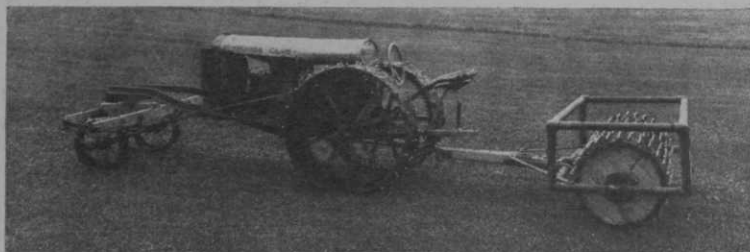
A pioneer team in power maintenance. The first Toro and the first spiked roller for fairway use. The latter built by Charley Erickson, veteran greenkeeper at Minikahda.
