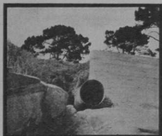
Scene of the 1929 National Amateur Championship matches . . . Pebble Beach course, Monterey County, Calif., is protected by Armco drainage, including this 36-inch stream enclosure of Armco Corrugated Iron Pipe under the 18th green.
