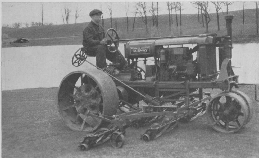
This new type of gang mower, designed for use with the FAIRWAY, is another compact unit that combines with the FAIRWAY in reducing maintenance expense on golf courses
