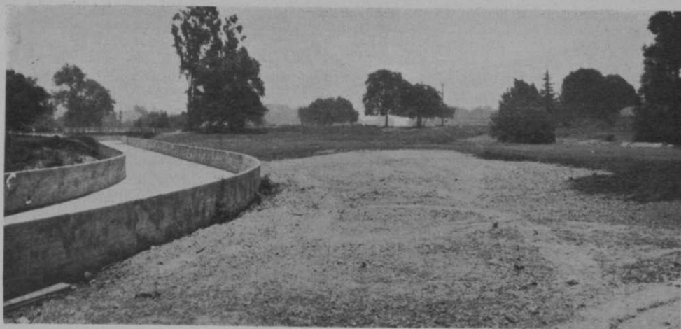
To prevent fairway erosion during the annual rainy season, this concrete flume has been built at the San Gabriel (Cal.) C. C. in the former river-bed. This view was taken during construction of the flume.
