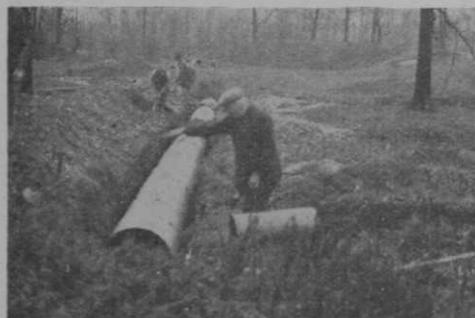
Bert Sheldon, greenkeeper at the Cleveland Country Club, superintending installation of Armco Perforated Pipe on his course.
