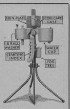
The Sure-Clean Washer will clean one to six balls at a time, and every mesh and dimple on the entire surface of the ball will be cleaned regardless of its condition.
