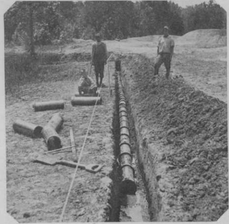
This drainage line, on the tenth hole, relieves the fairway of seepages along the hard-pan outcrops
