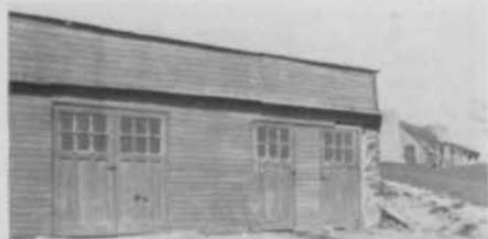
By using the basement of an old barn Westmoor got an equipment shed that is handy, inexpensive and practically concealed from the clubhouse by the side of a hill.
