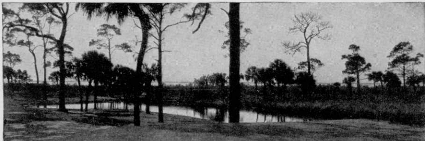
Above: A glimpse of Boca Ciega Country Club at St. Petersburg, Florida. A fleet of 16 International Trucks helped to make this development; from wilderness to finished course in 8 months.
