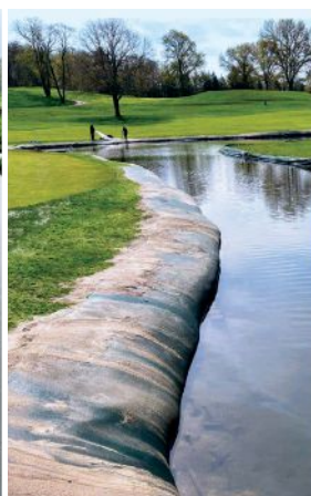
In this before, during and after series, a golf course creek’s banks is rebuilt with SOX and then grassed over.
