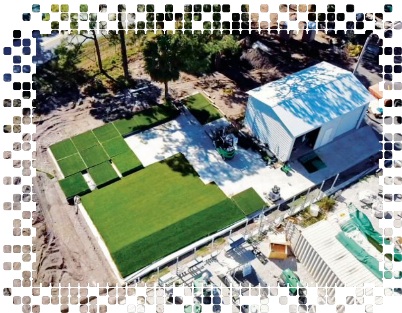
TGL's turf is grown on a concrete slab located 100 yards away from SoFi Stadium. The facility includes a storage building.
