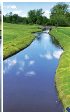
In this before, during and after series, a golf course creek’s banks is rebuilt with SOX and then grassed over.
